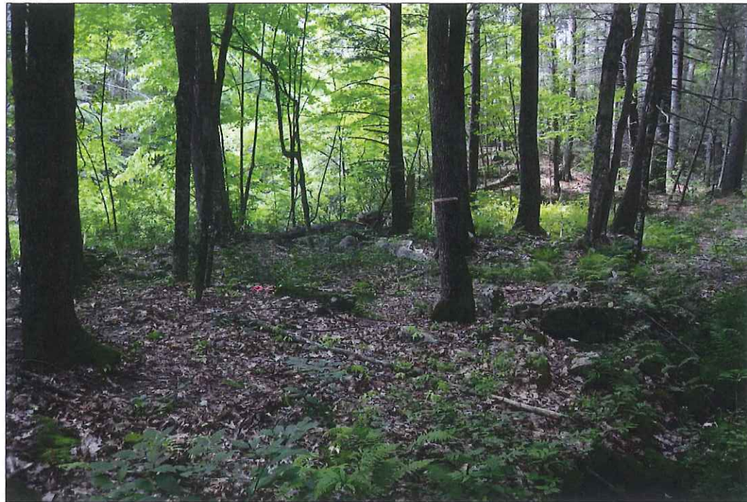
Figure 16. 2016 photograph of recti-linear stone foundation walls in the downstream reach below the dam (river left-north), view looking west.
