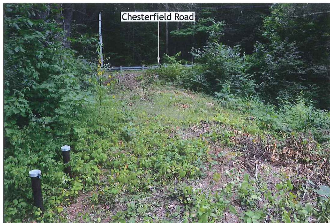
Figure 15. 2016 photograph of the proposed temporary access road (dam earth berm) off Chesterfield Road, view looking south.
