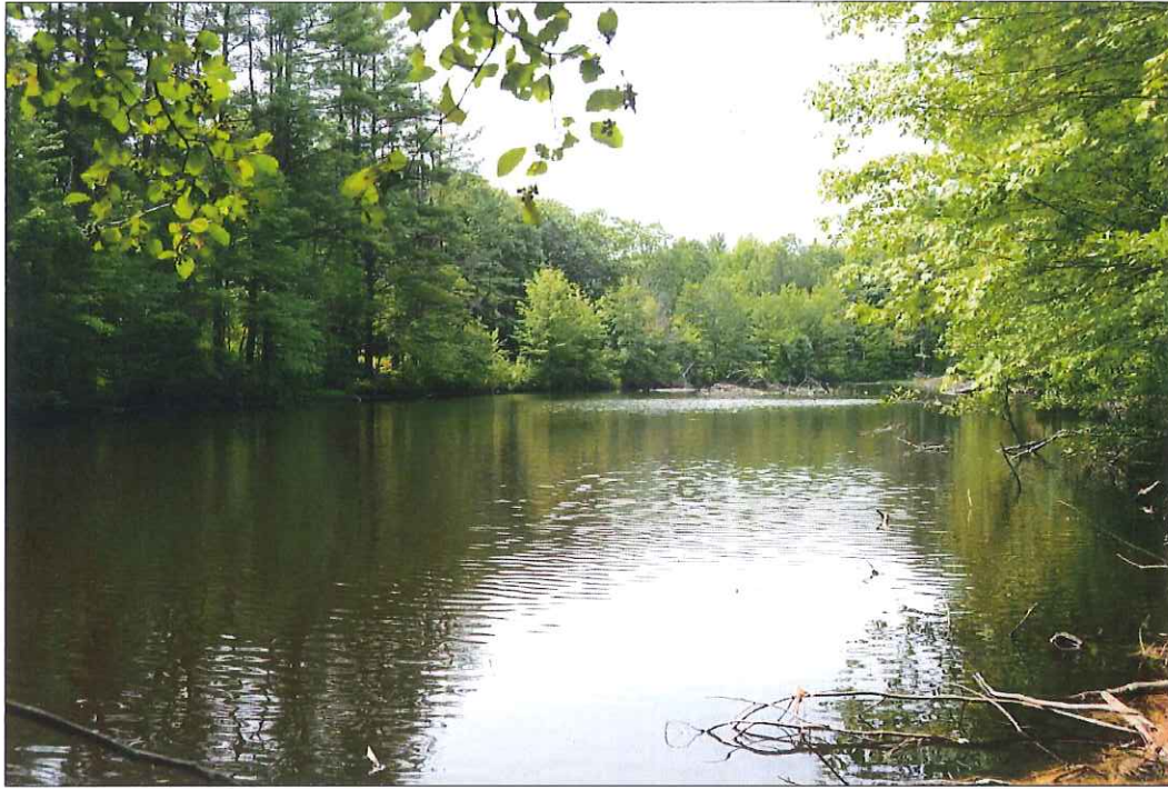
Figure 10. 2016 photograph of the Upper Roberts Meadow Reservoir, view looking upstream (south and west) from the dam.
