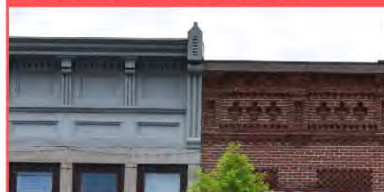
Cornice / Front Parapet Wall
